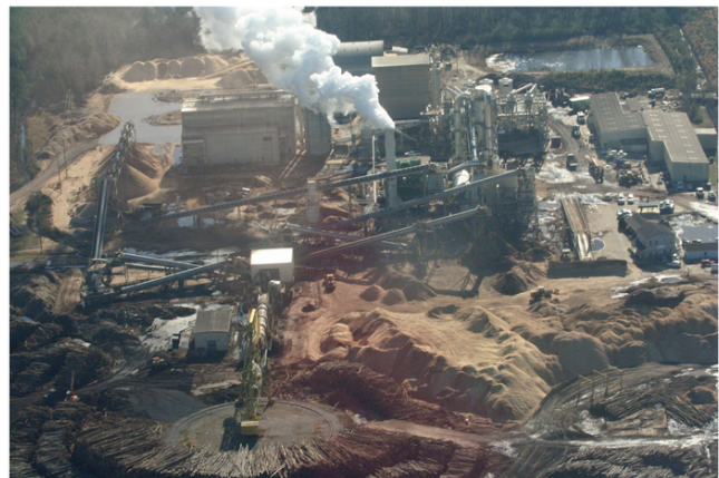
Enviva wood pellet plant in North Carolina
